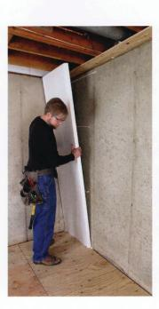
In most remodels, the foundation can't be insulated from the outside. Insulating the inside of a basement foundation with rigid expanded polystyrene sheets is an affordable alternative that reduces heat loss. For fire safety, the insulation board should be covered by drywall.
