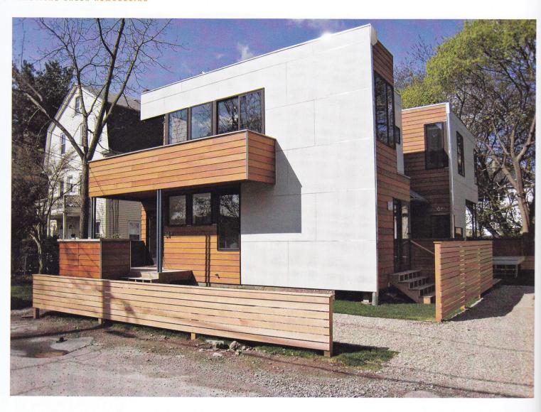
Rule-of-thumb load calculations don't apply. The high-performance building envelope of this remodeled duplex in Cambridge, Massachusetts, employs a continuous exterior layer of rigid foam insulation, resulting in heating and cooling loads 38% lower than conventional homes. The rightsized HVAC system is therefore smaller, less costly, and more economical to operate.
